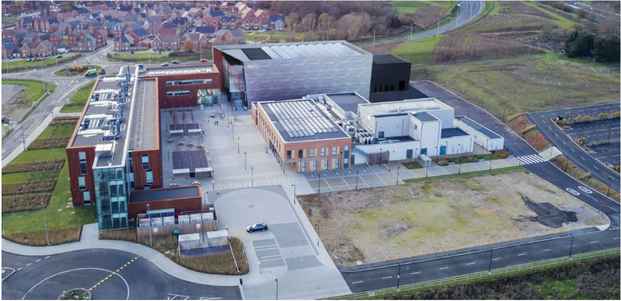
Figure 2: Image showing the TV studio building in the background linking to the existing Gateway building which is shown on the left of the image
