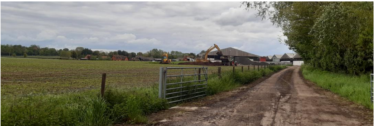
From site entrance on Dunt Lane
